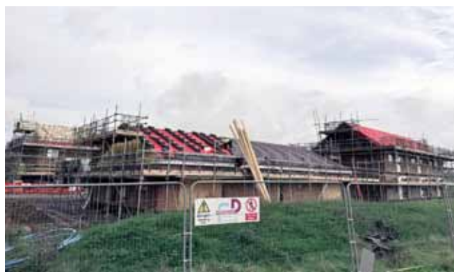
Roofing tiles going on at Reed Place in Rowde
