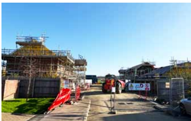
Building work well on its way at Reed Place in Rowde
