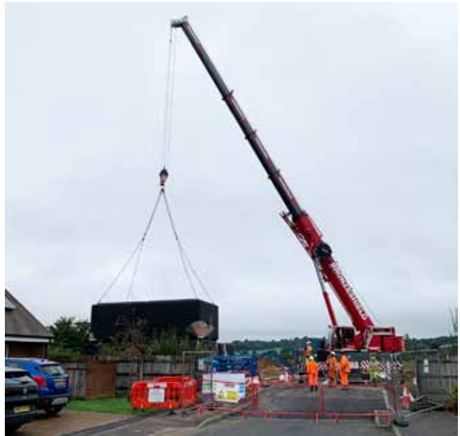
A ready-built home being craned onto the site at Reed Place in Rowde
