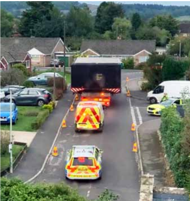
The ground floor section of a factory-built home arriving in Rowde
